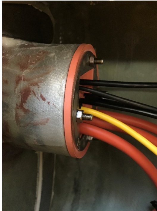
Figure 14 Guide showing gland nuts when tightened
